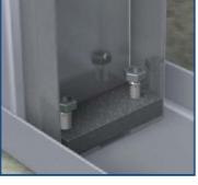
Attach 24" Midwall to the stud web with #12 screws fasteners through
